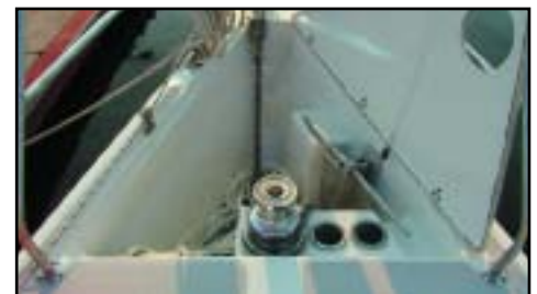
Anchor locker with cleat, place for second anchor and electric windlass with power up and down switches.
